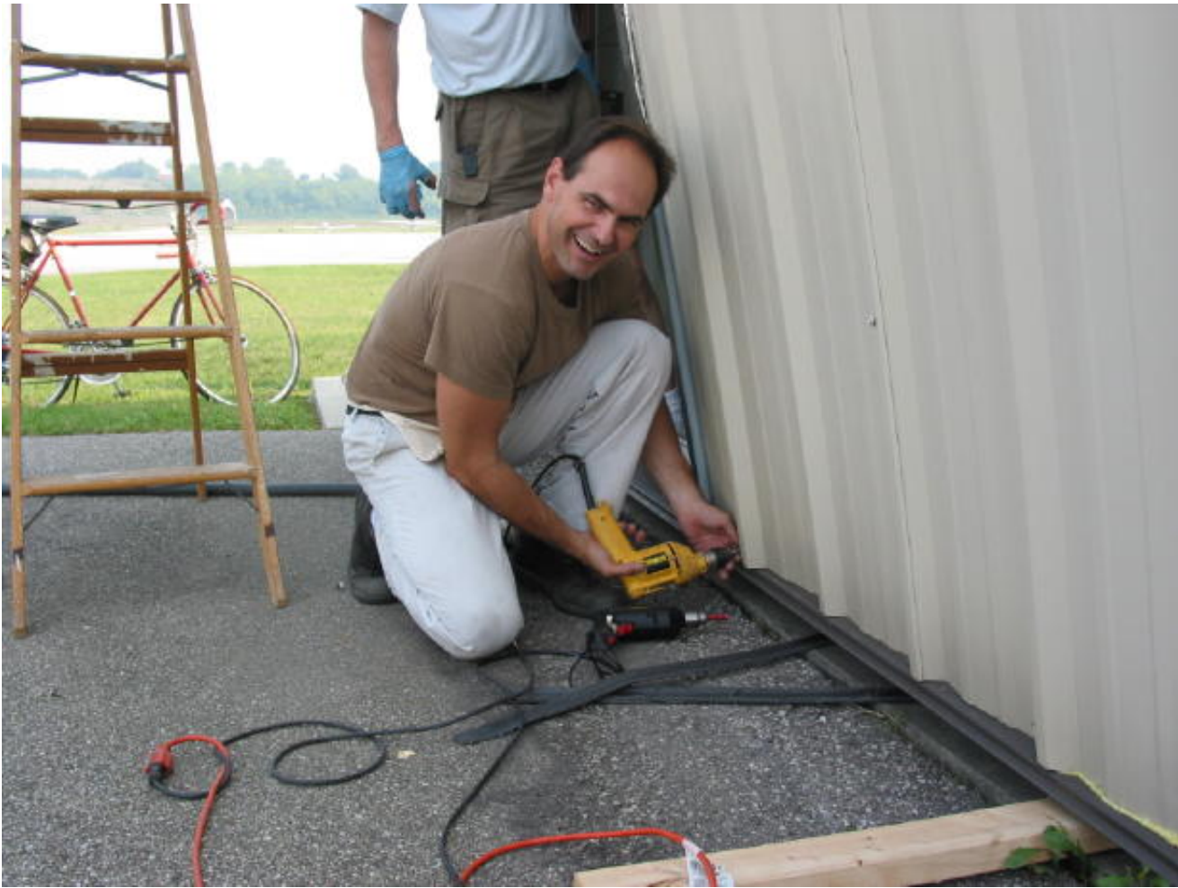
Note to readers, always look where you're drilling....
